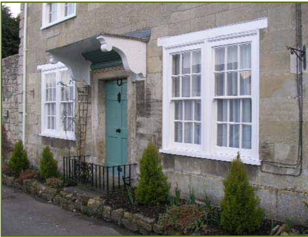
Figure 16. The use of the double sash, a characteristic of a number of buildings in the conservation area
