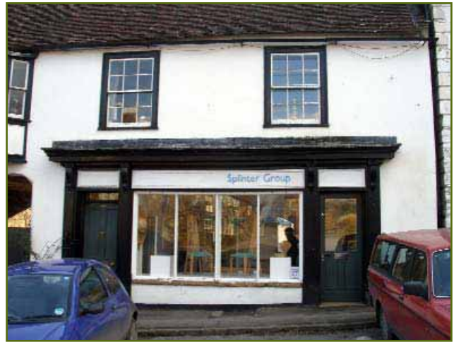
Figure 17. Good survival of nineteenth century shopfronts in the High Street
