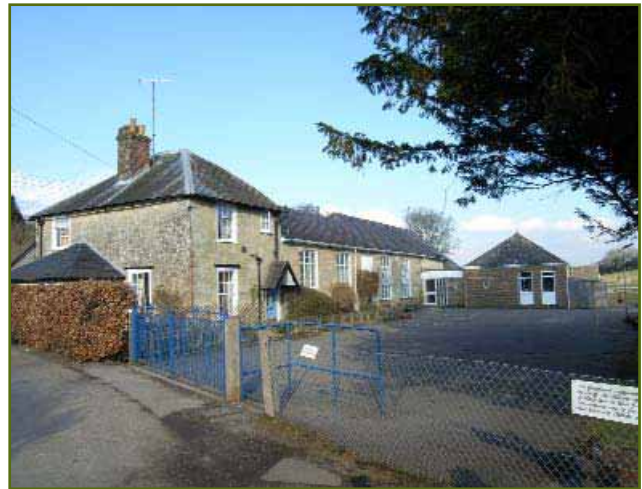
Figure 13. School House, late Georgian in overall character but with sashes set flush with the façade
